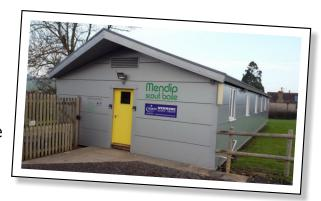
2014 insulated wall cladding replaced the original timber cladding, followed by a new insulated roof and the Bunk Room's fitting-out in 2016. Finally, in 2017, LED light fittings were installed throughout the building.
